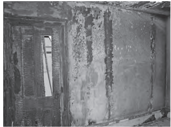
Figure 14. View northeast in small bedroom (107) where the fire started.
