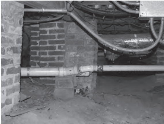
Figure 3. View west from beneath back porch. The gray mortar of mid-twentieth century alterations contrasts with the light mortar of one of the T-shaped piers, left of center, that were part of the original masonry.
