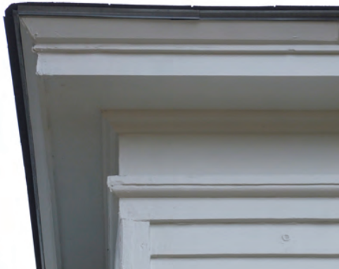
Figure 14. View of typical original exterior woodwork.
