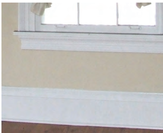
Figure 21. View of typical antebellum baseboard and window trim.
