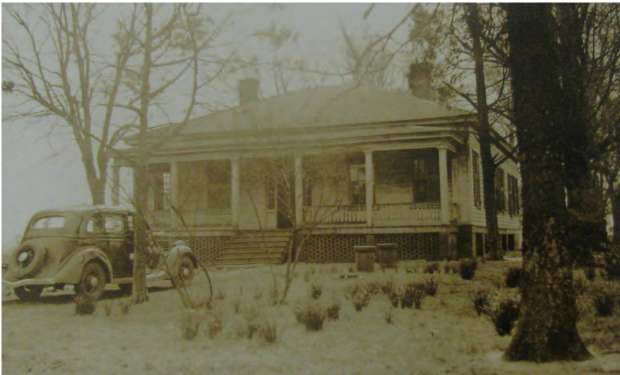
Figure 2. View of front of Dunlap House , probably taken around the time the government acquired the property in January 1935. (OCMU Collection)
