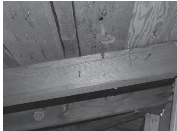
Figure 8. View of roof decking on west slope of roof, showing typical rafters and original 6" decking showing nails from original wood-shingled roofing. The narrow strips were used to create a solid wood deck for a standing-seam metal roof installed in 1938. At right is plywood decking used for repairs when the metal roofing was replaced with three-tab asphalt shingles in the last decade of the twentieth century.
