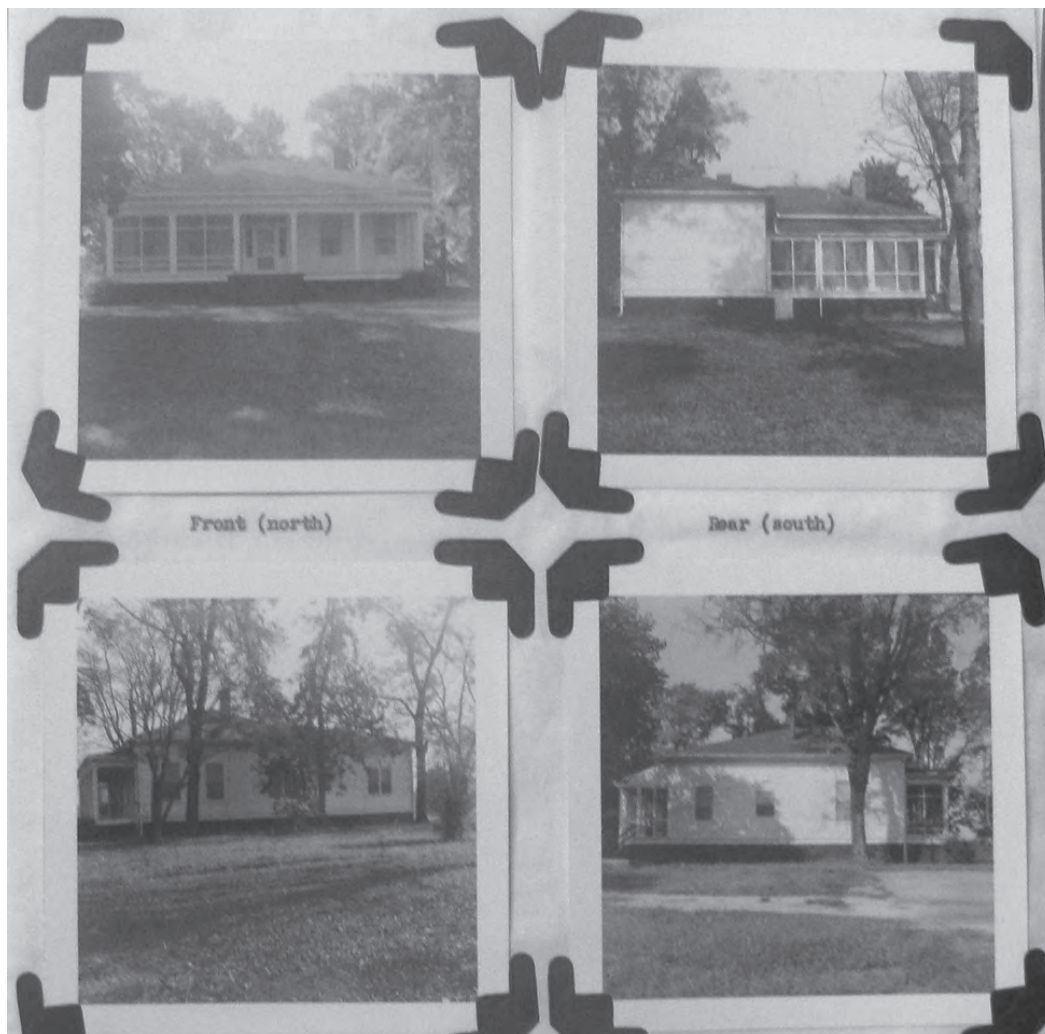
Figure 10. Four views of the house shortly after the 1952-1953 rehabilitation was complete. (OCMU Collection)
