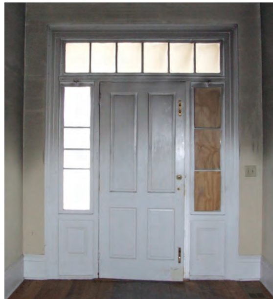
Figure 12. View of front door, transom, and side lights.
