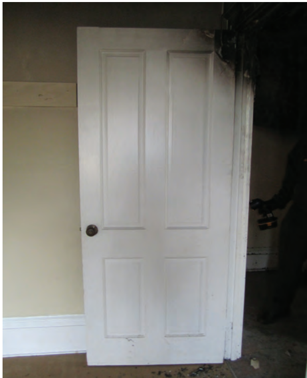
Figure 24. View of typical four-panel door.
