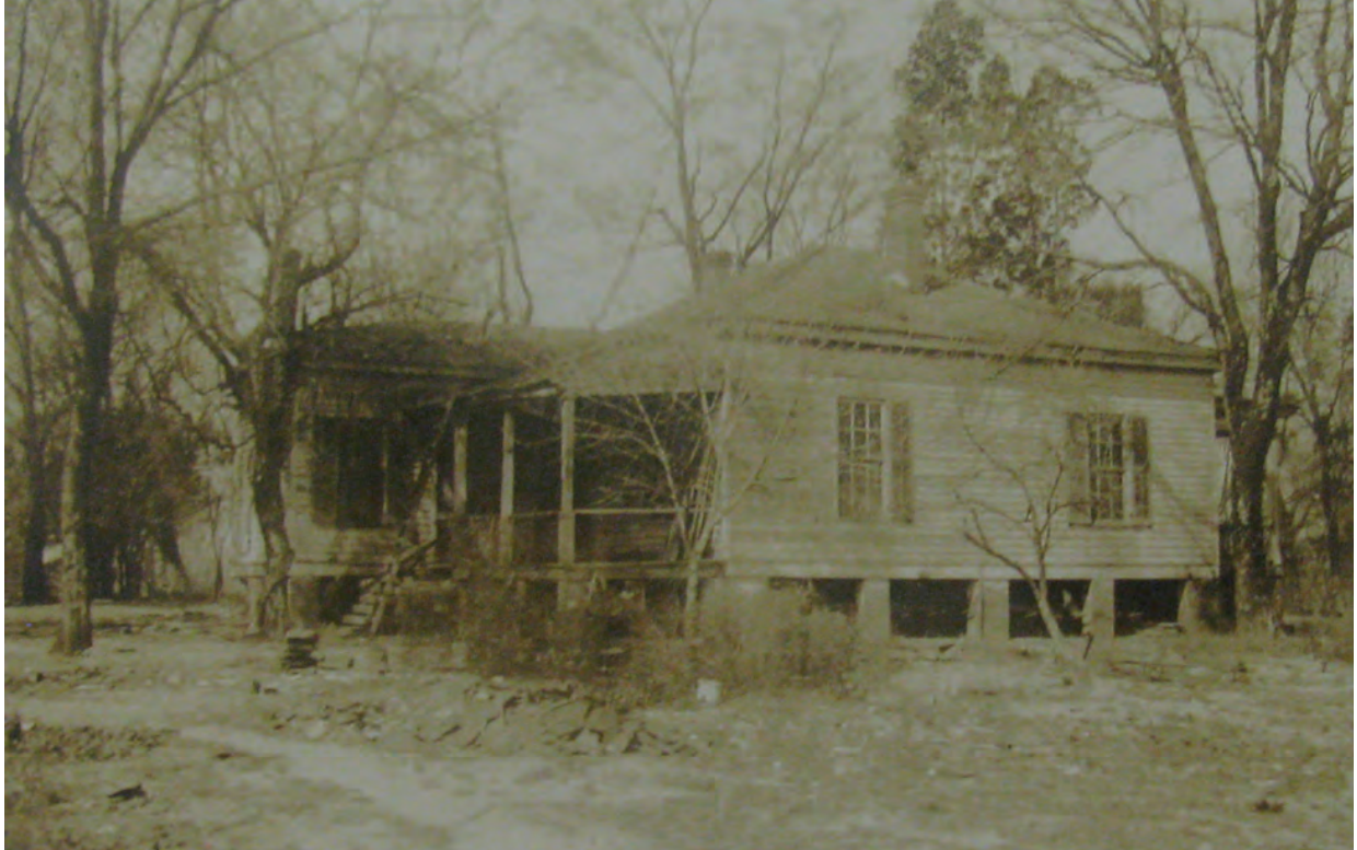
Figure 5. View northwest of Dunlap House, probably in 1935. Note that the old kitchen structure had already been removed by the time this image was taken. (OCMU Collection)
