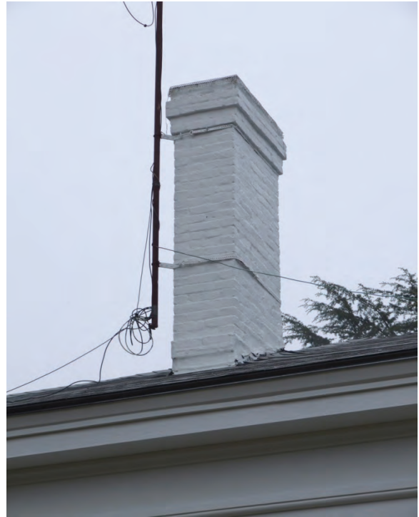
Figure 5. View of west chimney and part of attached television antenna.
