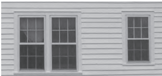
Figure 10. View of window openings created in 1952, all of which included a drip cap not present on the original window openings.
