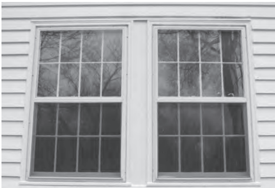
Figure 11. View of window opening at south end of Room 107, created in the last quarter of the twentieth century.
