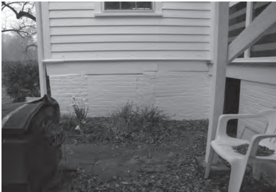
Figure 4. The anomalies in the foundation wall and skirt trim on the east side of the rear wing probably relate to the original configuration of the back porch. Beneath the present porch, a portion of the foundation is painted red, most likely after 1936 when part of the south foundation under the present kitchen was exposed.
