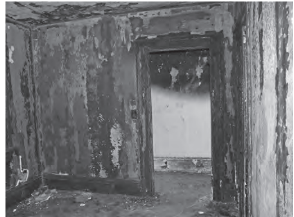
Figure 15. View west in small bedroom. All of the woodwork seen here, except for the baseboard in the hall, was charred beyond repair. The door in this opening was also destroyed.
