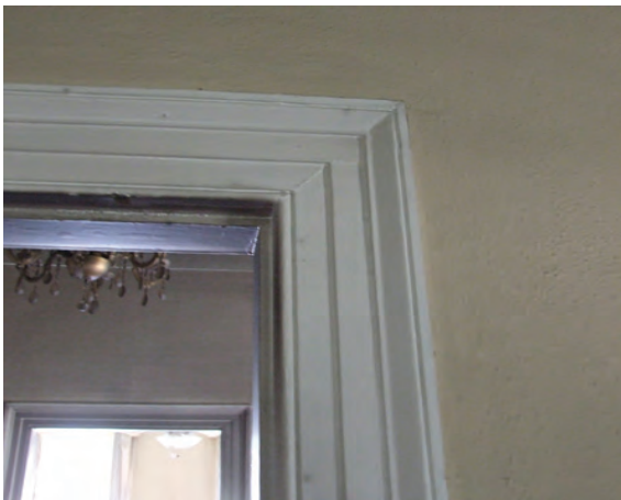
Figure 20. View of Living Room casing, typical of the original wood trim in the house.
