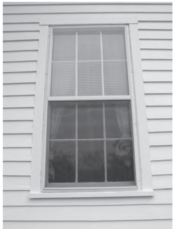
Figure 9. View of typical 1856 window opening.
