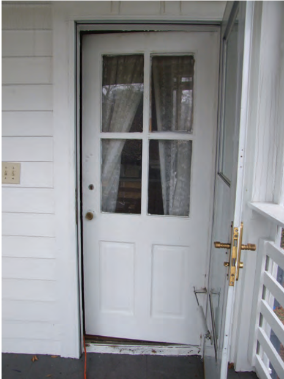
Figure 13. View of kitchen back door, installed in 1952.
